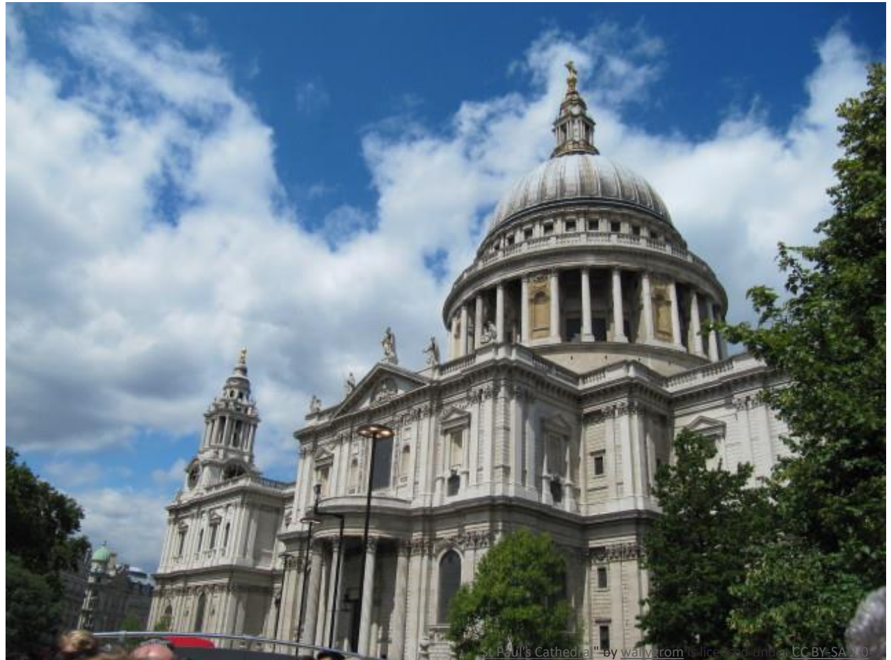
Figure 2.1: St Paul's Cathedral located on Ludgate Hill within the City.
