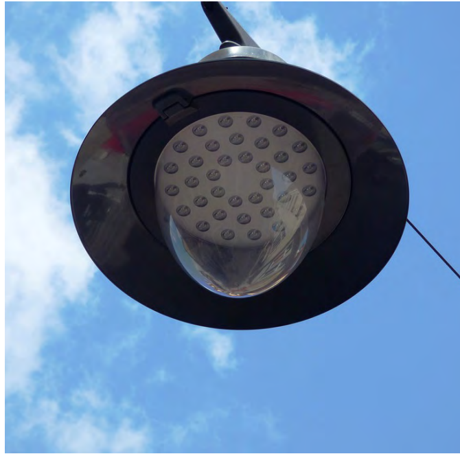
Unsympathetic LED retrofit of historical style lantern
