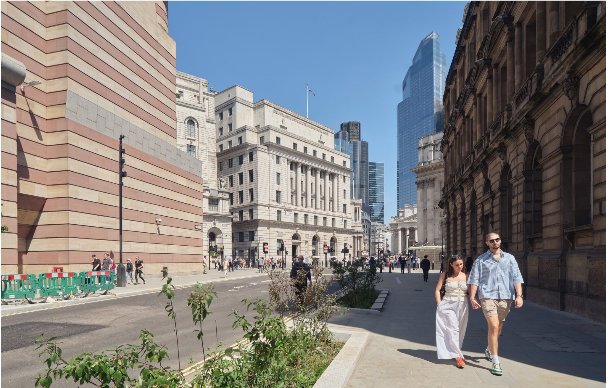
Bank Junction Junction: Rain gardens designed to capture surface water from the footway and the carriageway installed along Queen Victoria Street.
